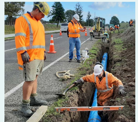
Stormwater pipelaying in Tasman Rd, Ōtaki. Courtesy Kāpiti Coast District Council.
